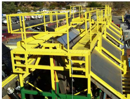
Figure 2: Genesis Rapid Dewatering System (RDS)
